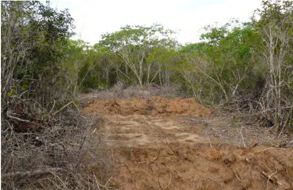
Figure 24. Prospecting cutline 'sealed off' using bulldoz- ers and cut branches, Palma area.
